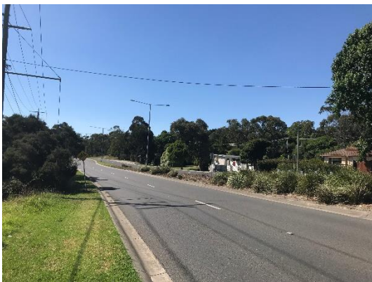
Figure 2.3: Swansea Road looking North (adjacent to site)
